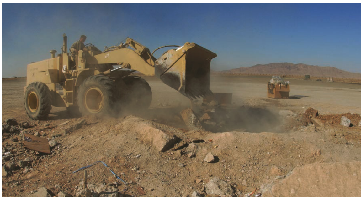
Photo by CPO Johnny Bivera, USN. Defense Imagery, VIRIN: 011227-N-2383B-508 Seabees of Naval Mobile Construction Battalion 133 fill bomb craters along the runway at Kandahar International Airport on 27 December 2001. The craters were created by Coalition forces during the initial phase of Operation Enduring Freedom.
