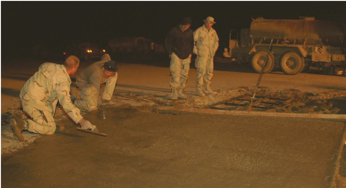
Photo by CPO Johnny Bivera, USN. Defense Imagery, VIRIN: 020108-N-2383B-516 Working through the night, Seabees of Naval Mobile Construction Battalion 133 smooth cement while repairing damage to the runway at Kandahar International Airport.
